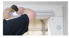
Attach the mounting bracket to a flat surface above the opening.
